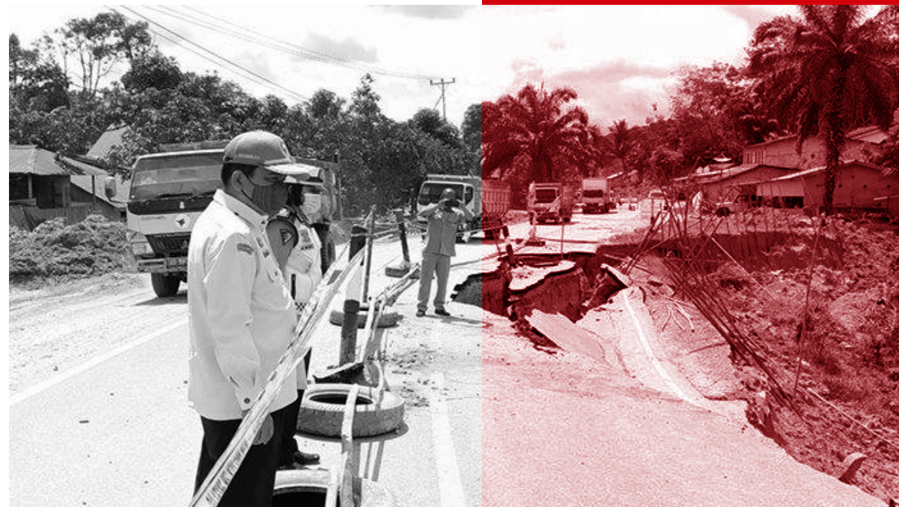
Photo 4. Erosion in the Tayan road as Impact of Toll Road Construction of Sosok – Tayan. 44
